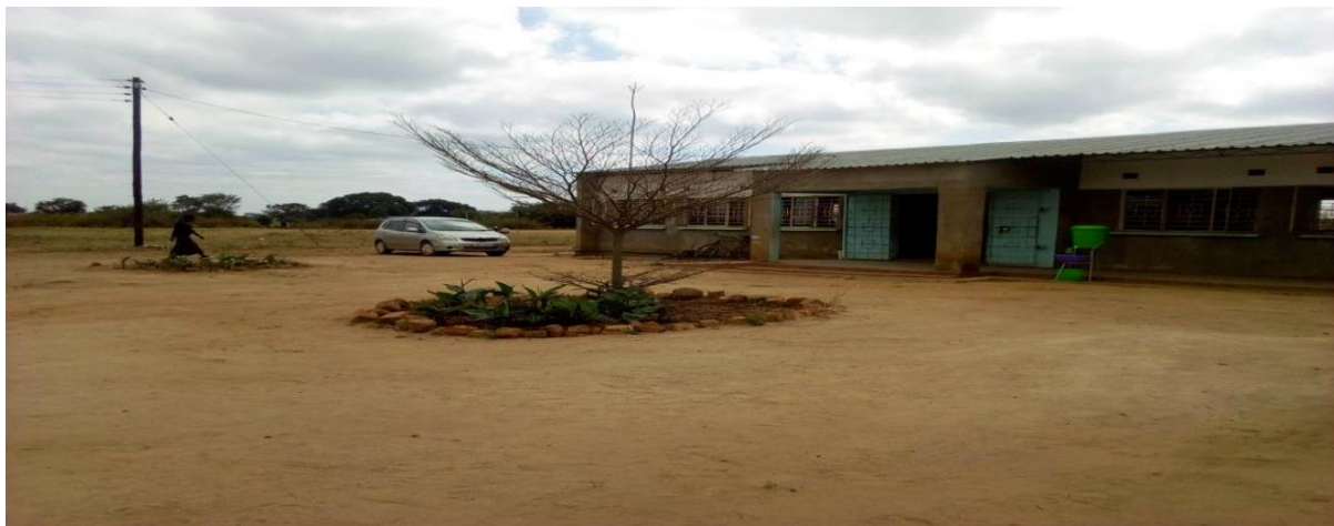
Katutulu Primary School in Kalulu forest
