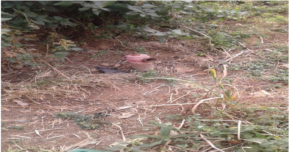
Figure 6.0: Water hydrant (Source: Author's field work, 2018)
